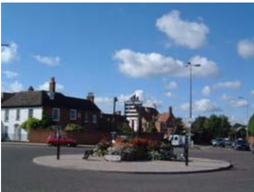
All works completed
